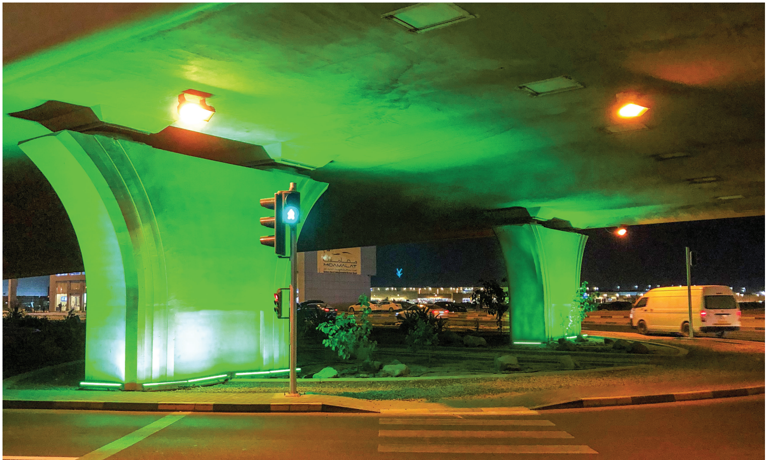
Project Name: Overpass Bridge Lighting , Ajman , UAE
