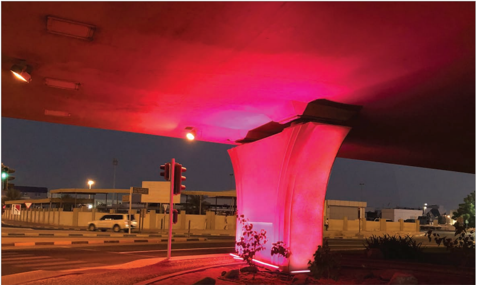
Project Name: Overpass Bridge Lighting , Ajman , UAE
